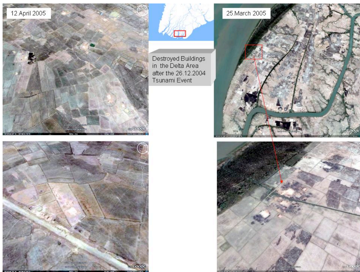
Fig. 5. Destroyed buildings in the delta area of the Irrawaddy River as documented by Google Earth images.
