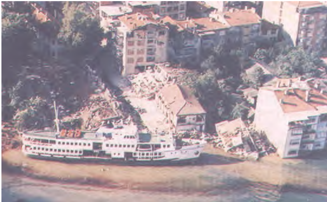
Figure 4: Extreme destruction from collateral ground liquefaction and subsidence (source: )
