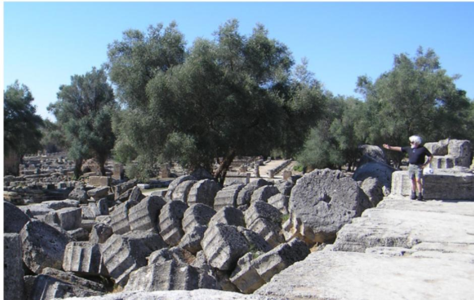
Figure 9. The directionality of failure of the Temple of Zeus massive Doric columns at Ancient Olympia provided clues as to intensity, maximum probable ground accelerations and source origin of the earthquake that caused their toppling (Photo G. Pararas-Carayannis).
