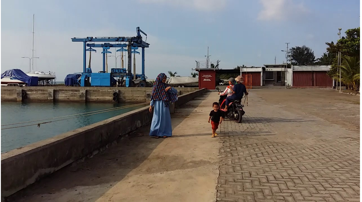
Figure 11 - The Marina Jambu tide gauge is in the center, the red building, before the installation of the IDSL.
