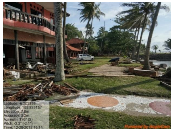
Figure 4. Debris in front of the building
