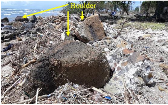
Figure 8. Boulders on top of the seawall in Batu Hideung Beach
