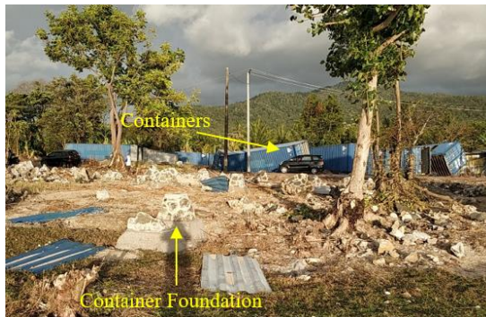
Figure 6. Container structure dragged by the tsunami
